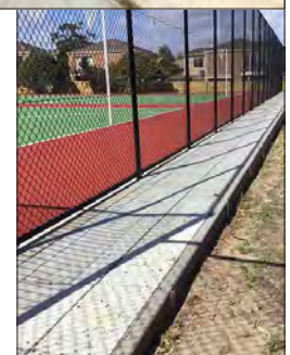
Support rails correctly spaced to allow mesh to be tautly fixed
