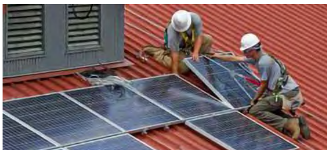
Workmen fixing solar panels on roof of industrial facility
