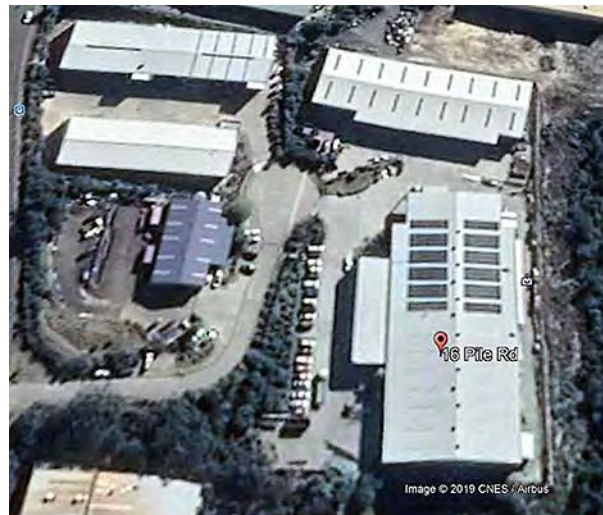
Protective Group 100KW Solar System in Somersby NSW
