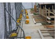
Photos show examples of braced temporary fencing with shade cloth attached
