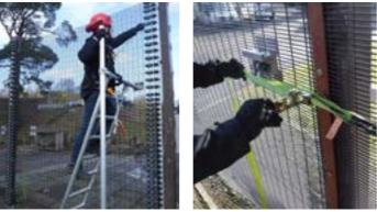
Working safely on 358 mesh using QAB safety brackets
