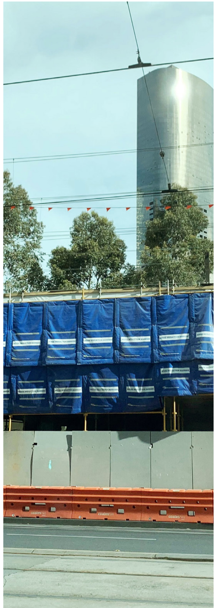
Noise abatement in Melbourne using acoustic barrier curtains
